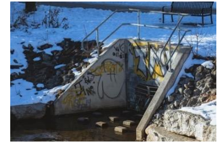
Storm and sewer
