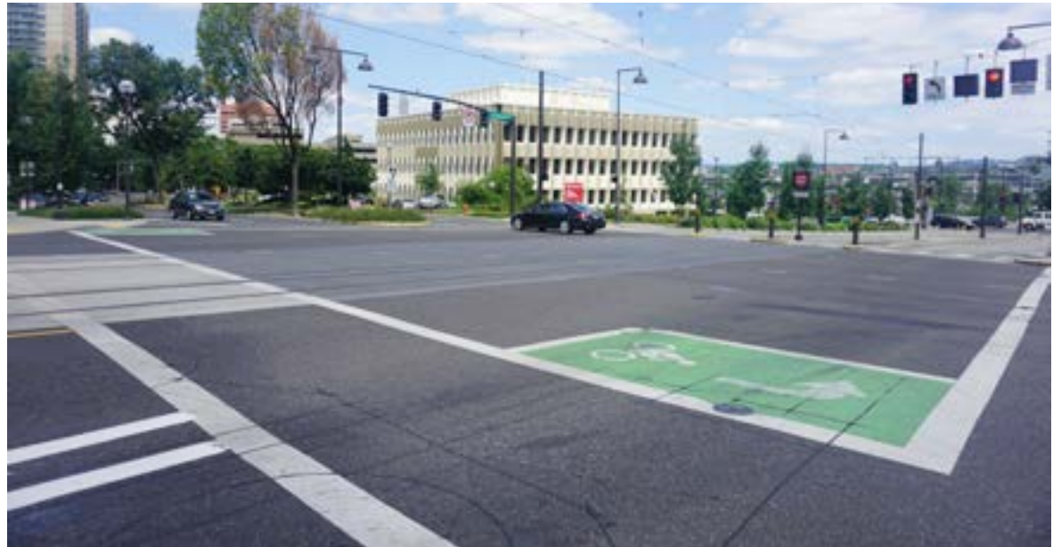
Top: Bicycle box; Bottom: Two-stage queue box
