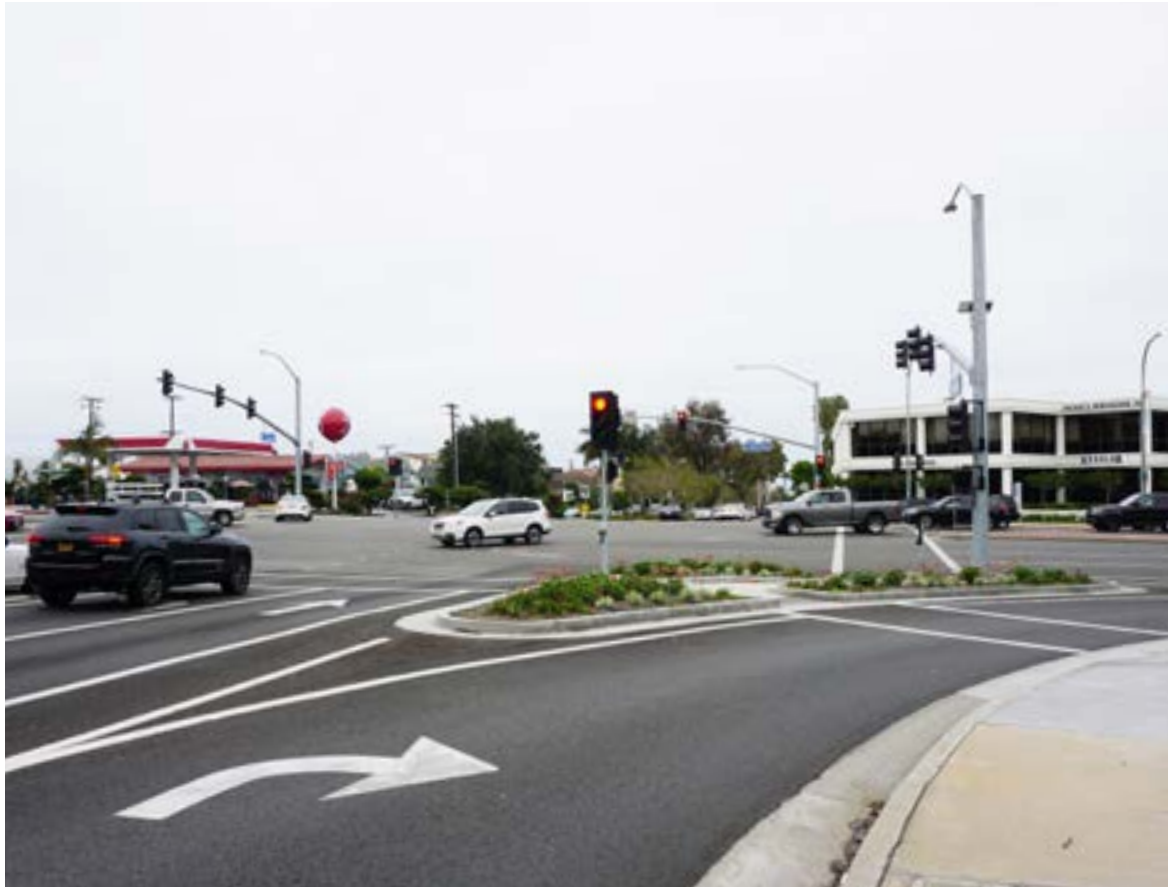
Channelized right turn
