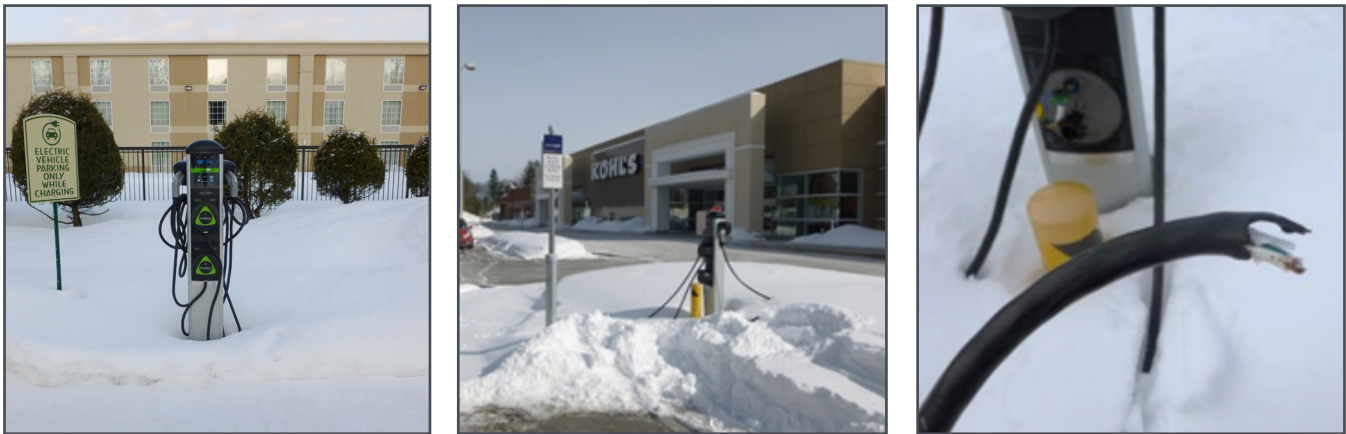
Figure 5. Snow accumulation can obstruct access to charging stations and snow plows can cause damage (right) Courtesy of Energetics Incorporated
