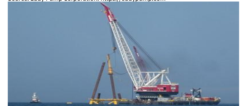
Source: DOSITS ( https://dosits.org/animals/effects-of-sound/anthropogenic-sources/pile-driving/ )
