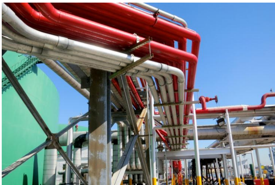
Figure 28. Electric Wiring Runs Along Elevated Conduit
