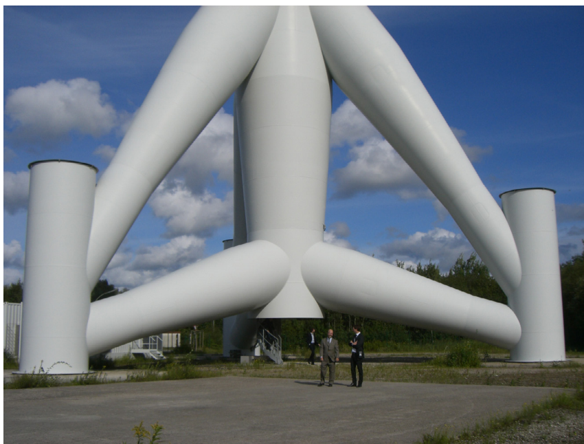
Figure 22. Tripod Substructure Used in 5-MW AREVA Multibrid Turbines Installed at Alpha Ventus near Bremerhaven, Germany
