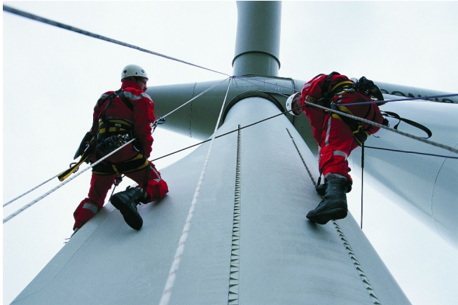
Figure 18. Siemens OSW Blade Repair
