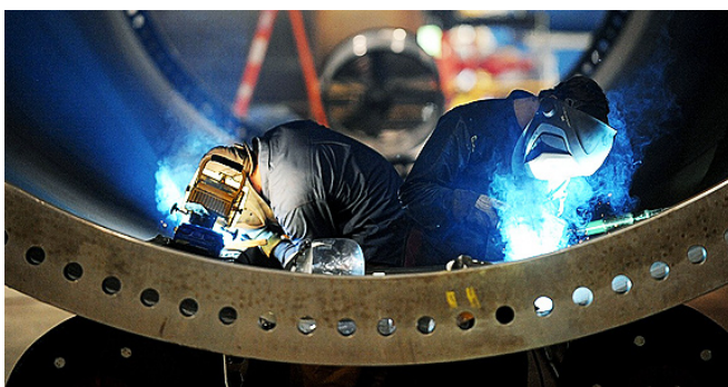
Figure 7. Ventower Welding Tower Flange
