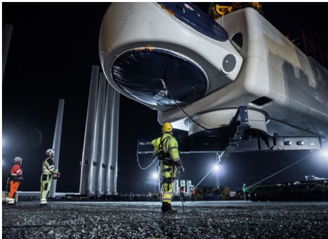
Figure 16. MHI Vestas Nacelle Arrives for Pre-assembly in Belfast for Orsted Energy's Burbo Bank Extension OSW Farm
