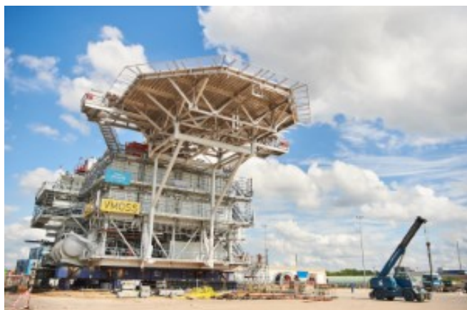
Figure 14. Veja Mate Offshore Substation
