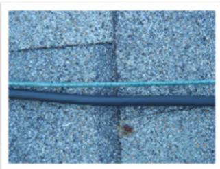
Photo 8 : Source circuit conductors in contact with roof: NEC 338.10, 334.30
