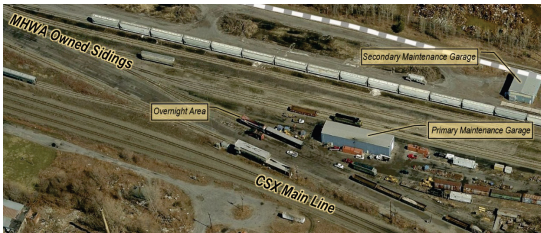
Figure 27. MSHA Utica Rail Yard
