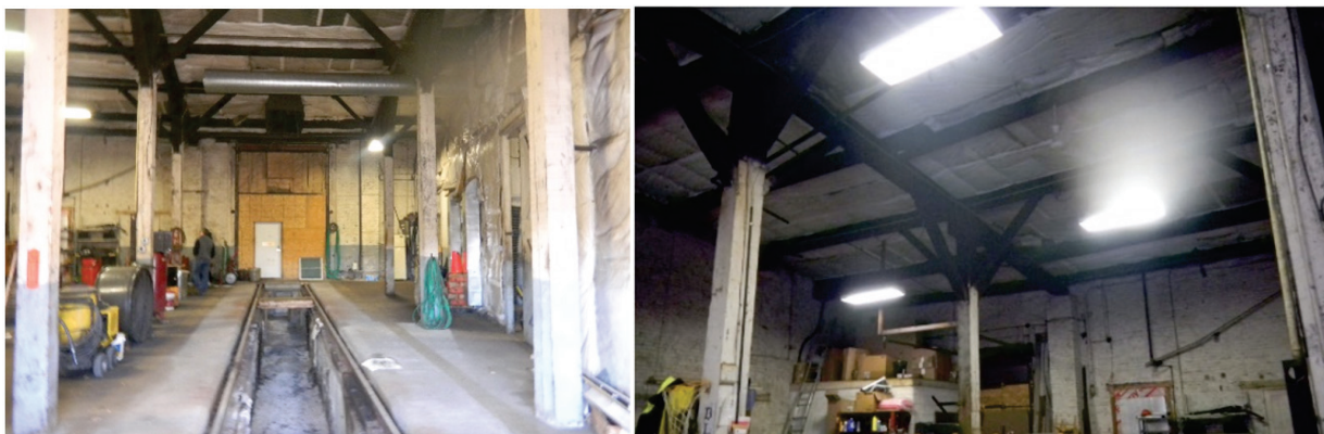
Figure 42. Existing Maintenance Facilities
