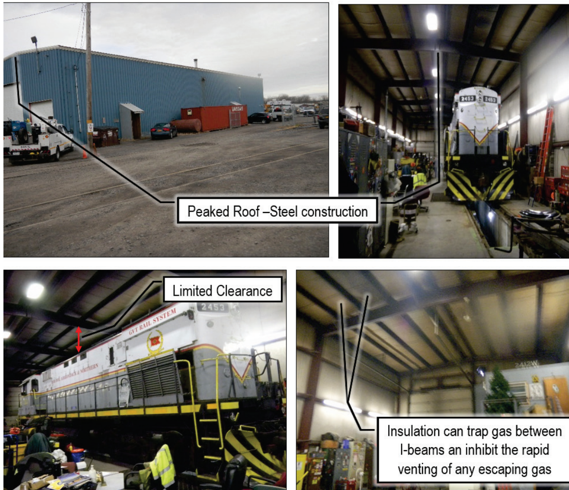
Figure 19. Utica MHW Maintenance Facility Considerations for CNG
