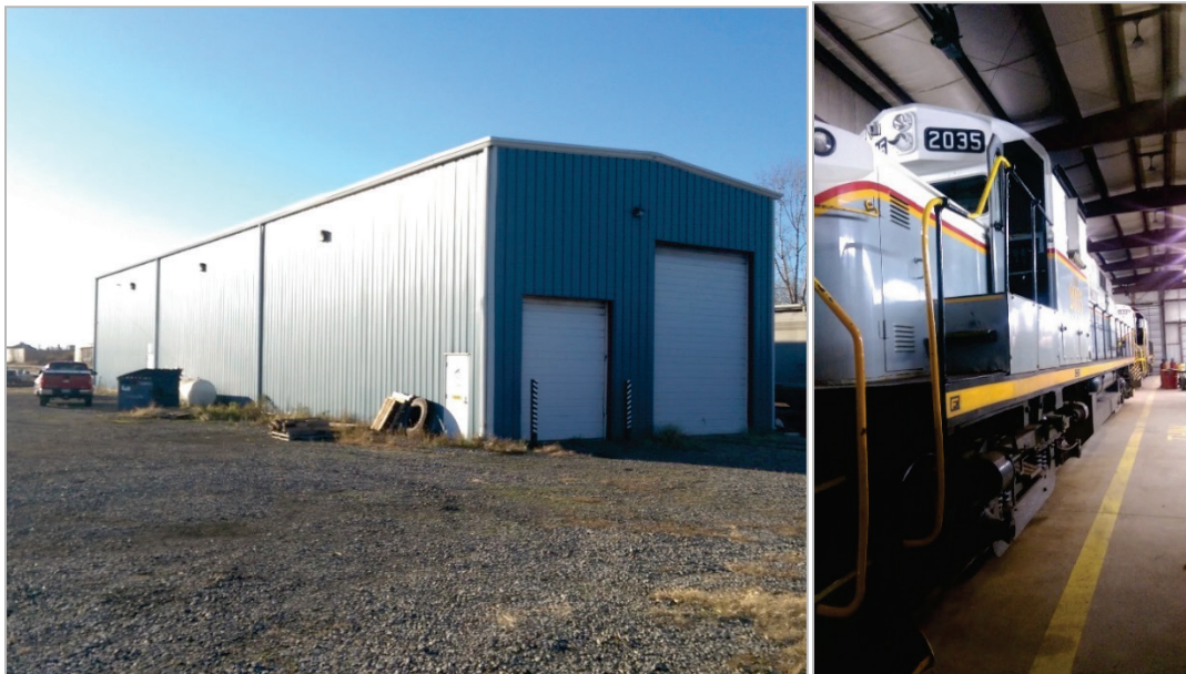
Figure 44. Falls Road Railroad Maintenance Facilities in Lockport
