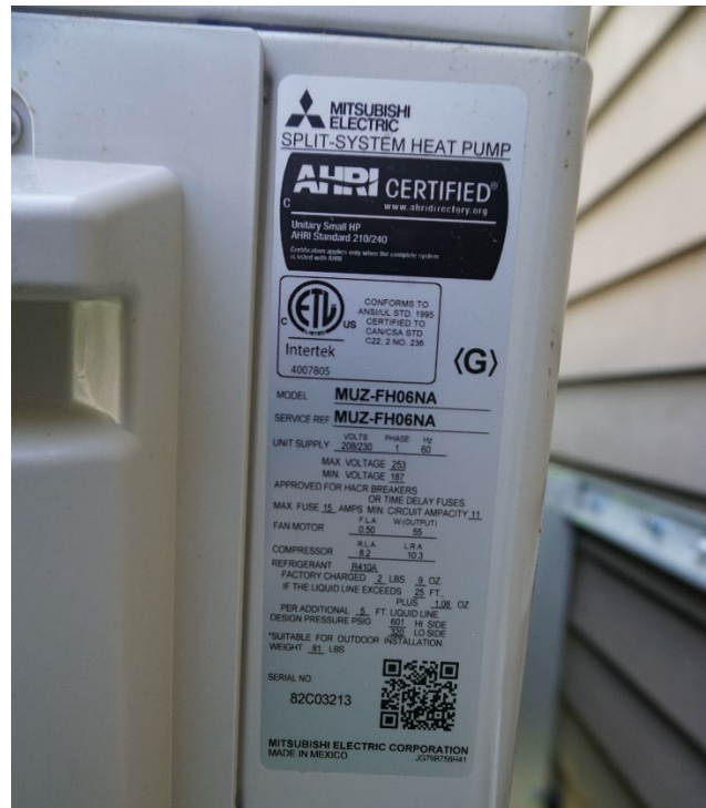
Smaller Outdoor Unit (Model #MUZ-FH06NA)
