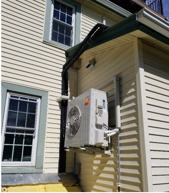
Larger Outdoor Unit (Model # MUZ-FH18NA2)
