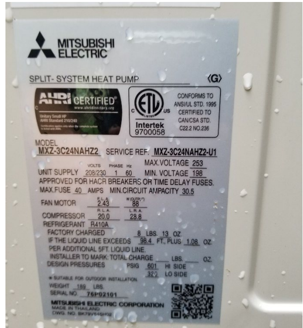
1 of 2 Outdoor Units - Nameplate Model #MXZ-3C24NAHZ2
