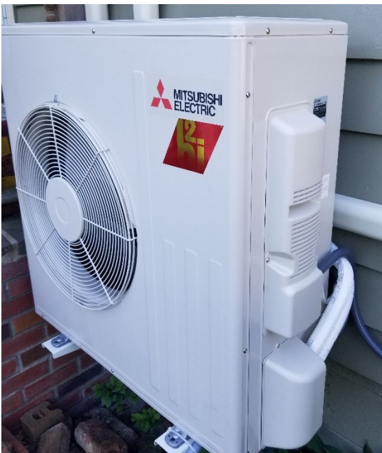
Larger Outdoor Unit (Model # MUZ-FH18NA2)
