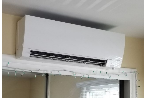
One of Five Indoor Sections (Bedroom)
