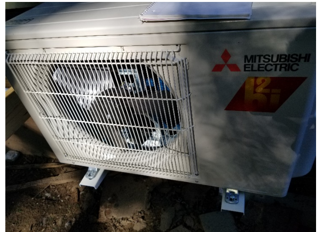
1 of 3 Smaller Outdoor Units (Nursery - Model #MUZ-FH06NA)
