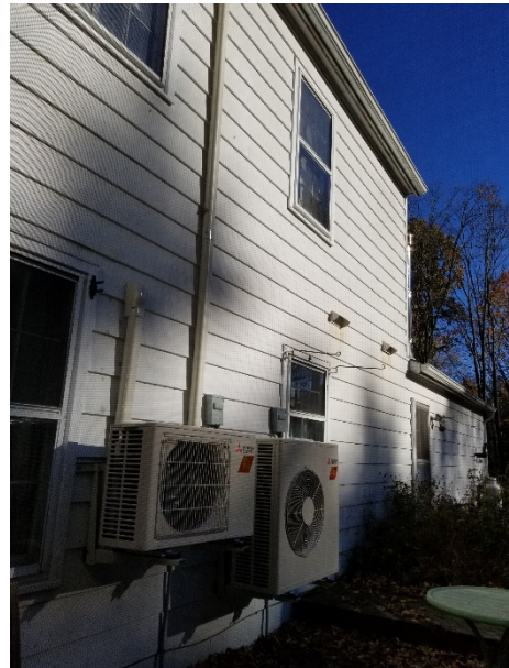
One Model MUZ-FH12NA (Left) One Model MUZ-FH18NA (Right)
