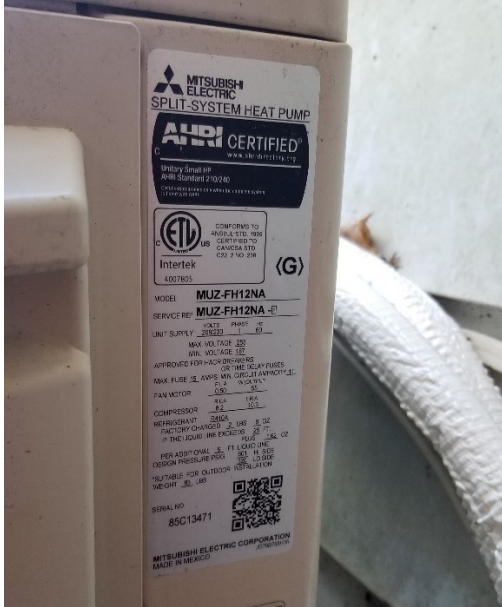
Outdoor Unit (Model #MUZ-FH12NA) Side of Home Outdoor Unit (Model #MUZ-FH12NA) Side of Home
