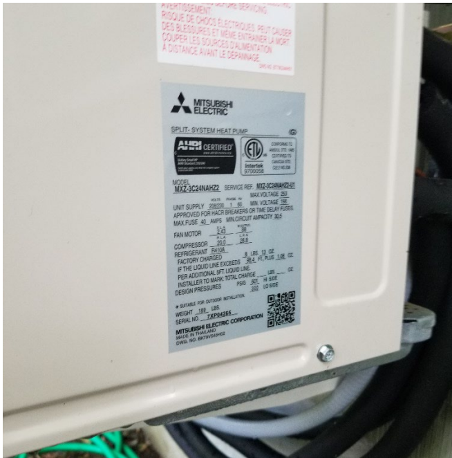
1 of 2 Outdoor Units - Nameplate Model #MXZ-3C24NAHZ2
