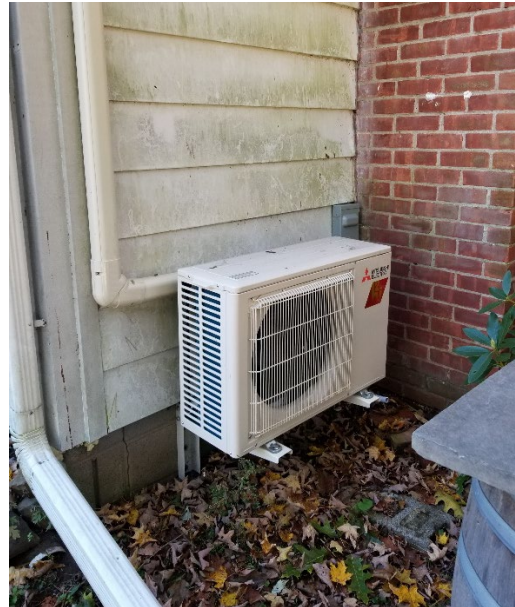
Outdoor Unit (Model #MUZ-FH12NA) Side of Home Outdoor Unit (Model #MUZ-FH12NA) Side of Home
