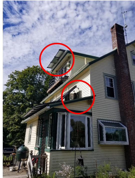
Smaller Outdoor Unit (Model # MUZ-FH06NA)
