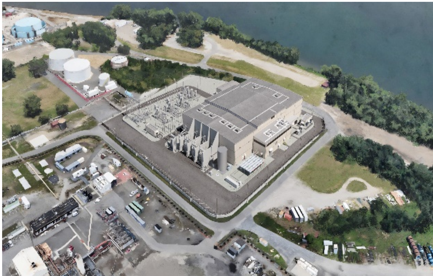
(Champlain Hudson Power Express Celebrates Start of Construction on Converter Station; Announces First Funding Recipients for Green Jobs Training Fund, n.d.)
