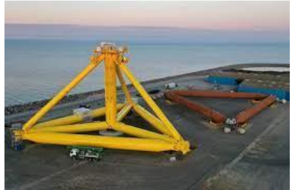
TetraSpar foundation components manufactured at the facilities of the Danish wind turbine tower manufacturer Welcon and transported to the port of Grenaa.
