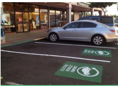
IMAGE 2. MILILANI, HI THE EVSE IS MOUNTED ON AN EXISTING POST AS TO NOT SHORTEN THE PARKING SPACE OR INTERFERE WITH PEDESTRIAN ROUTES.
