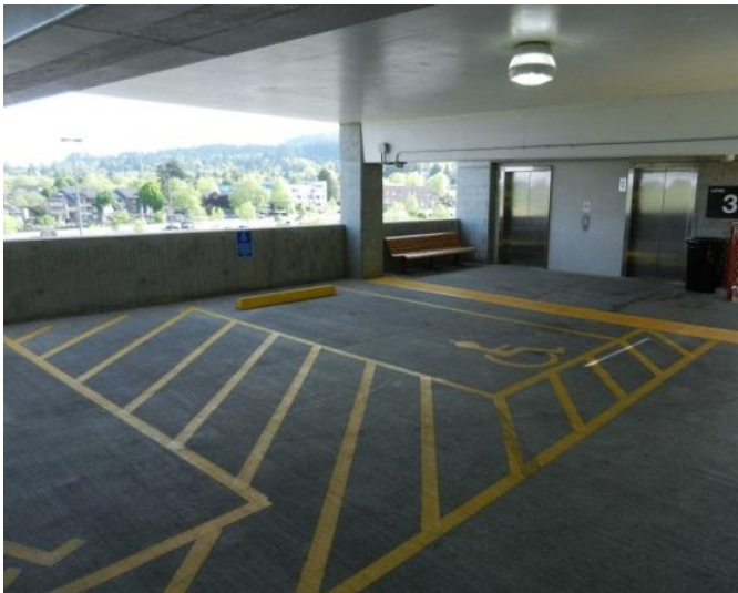
Existing ADA-compliant parking near elevators
