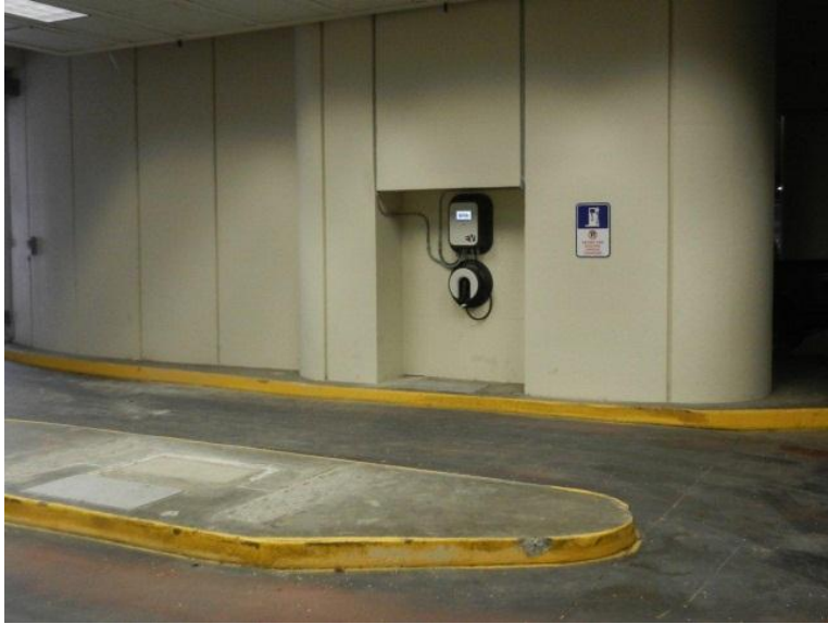
Former drive-up ATM converted to EV charging
