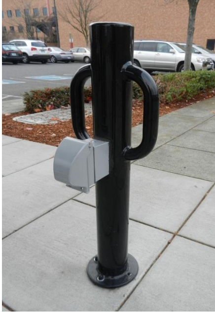
Level 1 EV supply equipment
