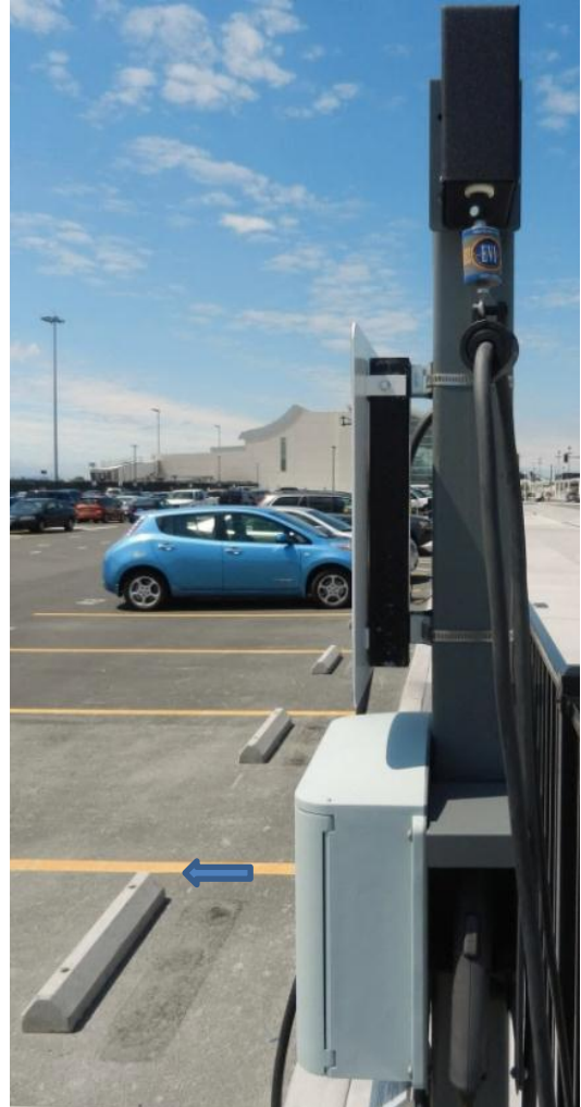
Moving wheel stops back can prevent vehicles from damaging EV supply equipment
