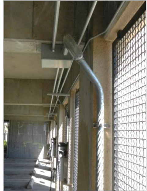
Ceiling-mounted conduit located near wall
