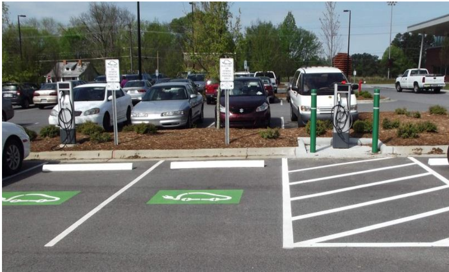
EV supply equipment placed in landscaping at Durham NC's south regional library (Photo courtesy of Robert Shuler, North Carolina Department of Insurance).
