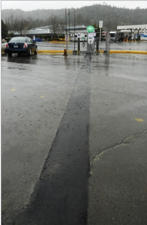
Trenching long distances to install electrical conduit raises costs
