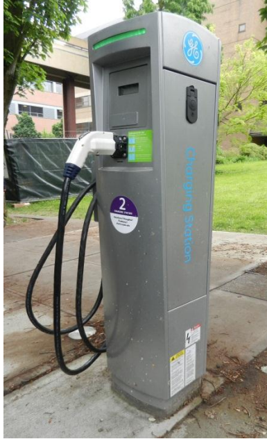
Level 2 EV supply equipment
