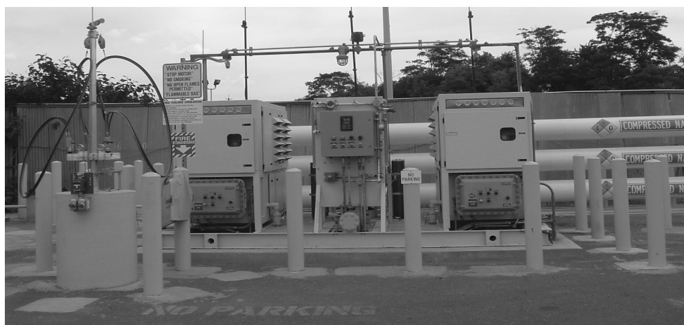
Figure 23. Manhattan Beer compressed natural gas fast-fill fueling infrastructure
